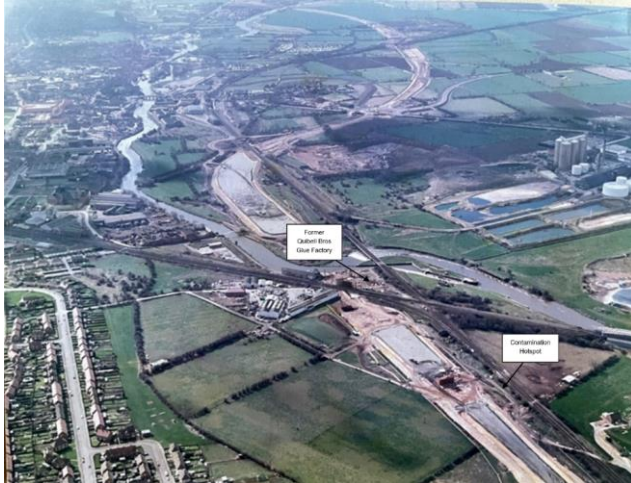
Photo 9-1: Contamination hotspot aerial photograph from construction of existing A46 road
